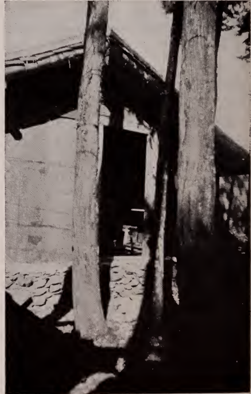
CHARCOAL STORAGE ROOM CONVERTED INTO MUSIC ROOM
